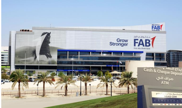
Headquarters Business Park, Abu Dhabi
